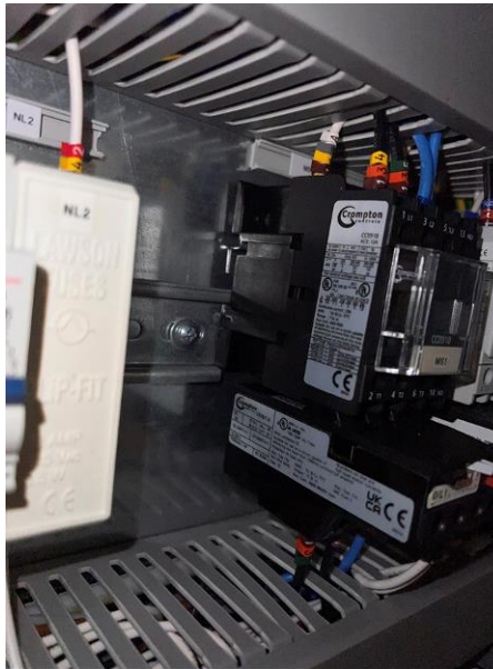
Replaced Contactor & Overload (MS1)
